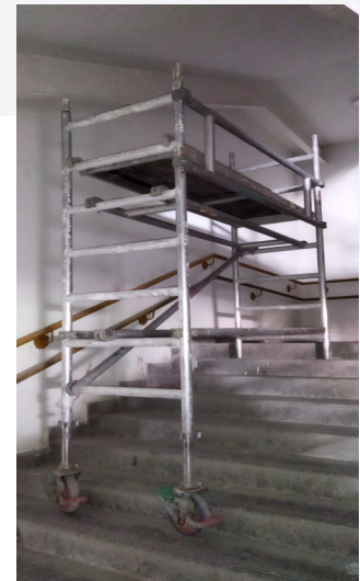
Scaffolding on Stairs
